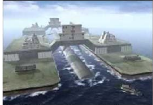
The 54,000 tunnel sections would be transported by a specialized ship called an immersion pontoon, then lowered into place.
